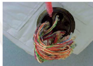
Fig. 2. Closure 31B - Applying Sealant.
