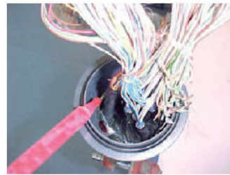
Fig.4. Closure 31J - Applying sealant.
