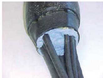
Fig.3. Closure 31J prepared for sealant
