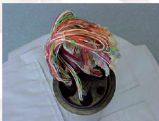
Fig. 1. Closure 31B prepared for sealant
